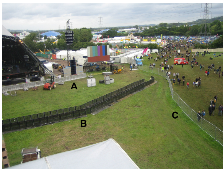
Fig. 23-2 - An example of a Primary (silver, A) and Secondary (black, B) barrier lines being installed with block-and-mesh (C) being used to delineate public and working areas. Photo courtesy of The Event Safety Shop, LTD.
