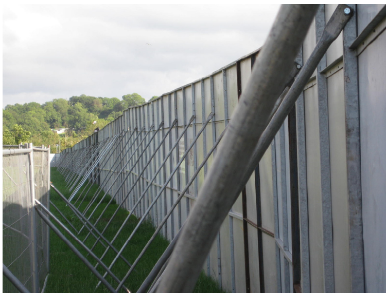
Fig. 23-4 - Solid temporary fence panels showing diagonal bracing. This is a pedestrian barrier used to channel queue lanes – perfect when no sideways pressure is anticipated. Photo courtesy of The Event Safety Shop, LTD.
